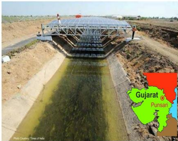
Fig 1.3.5 Canal solar power
